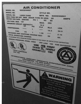
Fig. 7.5 A/C Data Plate
